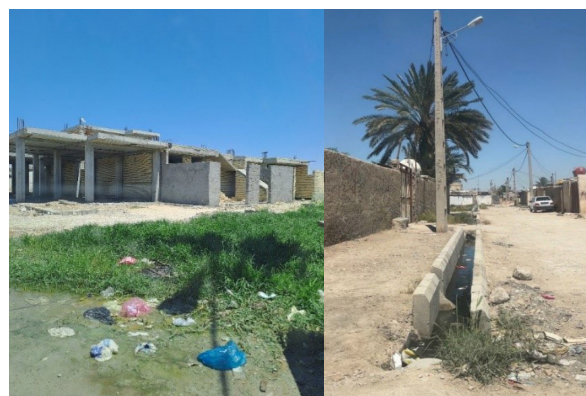
Fig. 1. Images of the neighborhood, the incomplete Housing Foundation building, improper waste collection, and inadequate basic and superstructure infrastructure. Source: Authors.
