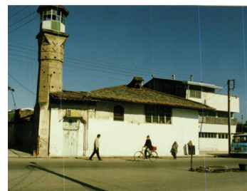
Fig. 30. Plan and Images of Doroodgar Mosque and Minaret, Babil. Source: Registration Dossier in the list of national monuments of Iran, General Directorate of Cultural Heritage, Tourism and Handicrafts of Mazandaran Province.
