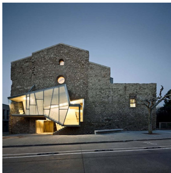
Fig. 8. Saint Francis Church. Source: www.archdaily.com.
