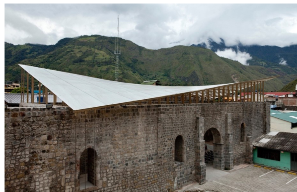
Fig. 7. Baños Church. Source: www.archdaily.com.
