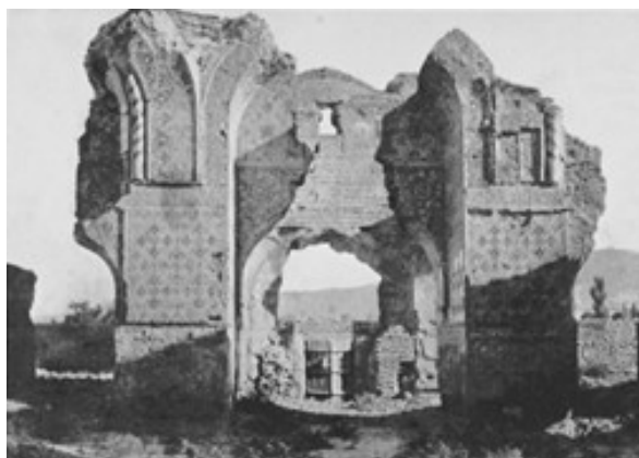
Figs. 13. The state of the mosque after the destructive earthquake. Source: Archive of the General Department of Cultral Heritage of East Azarbaijan Province.
