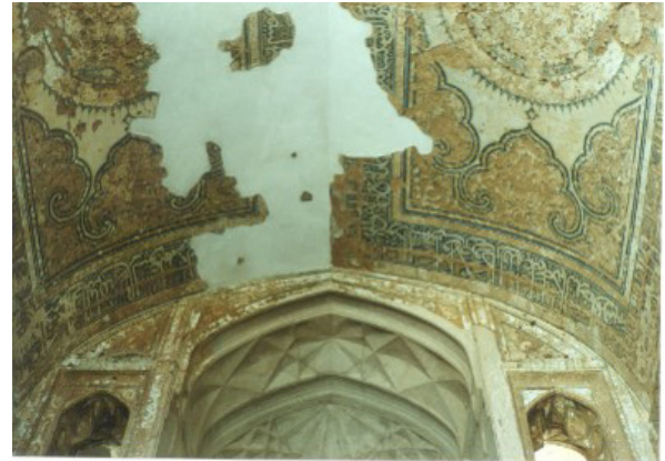
Fig. 4. Painting decorations under the arch of the dome chamber iwān. photo from the Cultural Heritage Department file.
