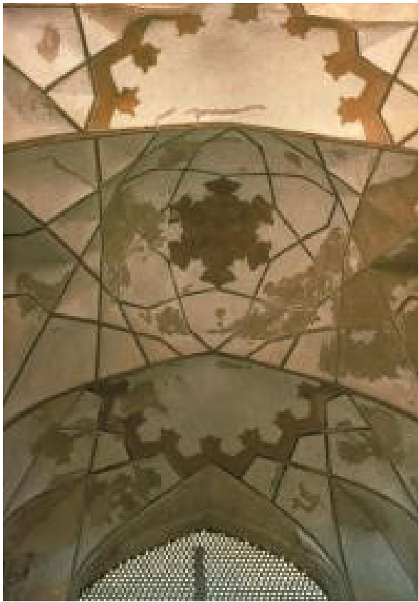
Fig. 5. Decorations on the ceiling of the dome chamber. photo from archnet.org.
